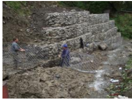
2013: Special Gabions built to seal the hill
