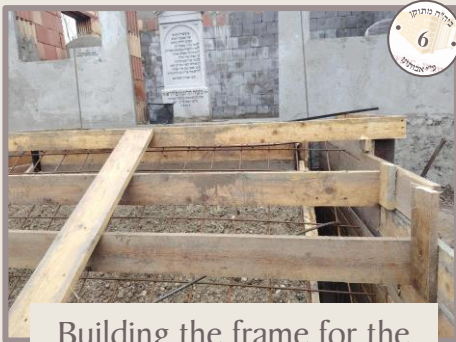
Building the frame for the steps to the Ohel entrance
