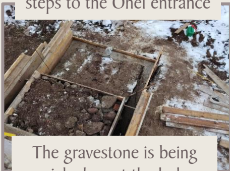
Building the frame for the steps to the Ohel entrance
