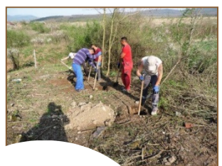
Preparing the foundations
